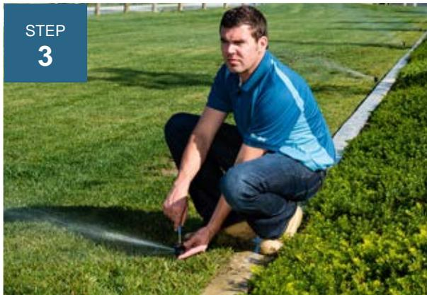
Walk through each station on the controller, checking for proper operation of the zone. Check for proper operating pressure (low pressure indicates a line break or missing sprinkler), proper rotation and adjustment of sprinkler heads, and adequate coverage. Check and clean filters on poorly performing sprinklers. Adjust heads to grade as necessary.
