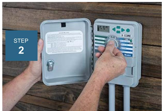
Verify the proper operation of each station valve by manually activating all zones from the controller.
