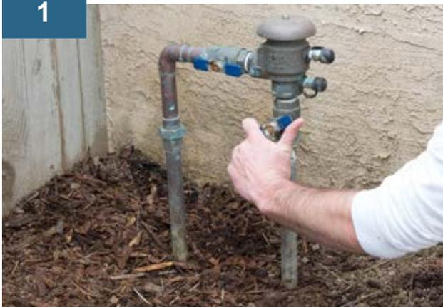
Open the system main water valve slowly to allow pipes to fill with water gradually. If these valves are opened too quickly, sprinkler main lines are subjected to high surge pressures, uncontrolled flow and water hammer, which may cause them to crack or burst.
